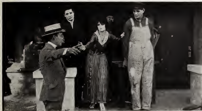
The Newlyweds in Bad
